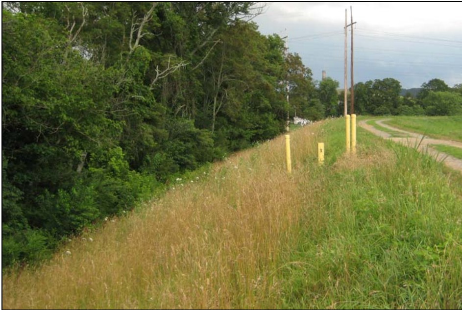
Photo 1. Well Maintained Embankment Crest, Showing Heavy Vegetation
