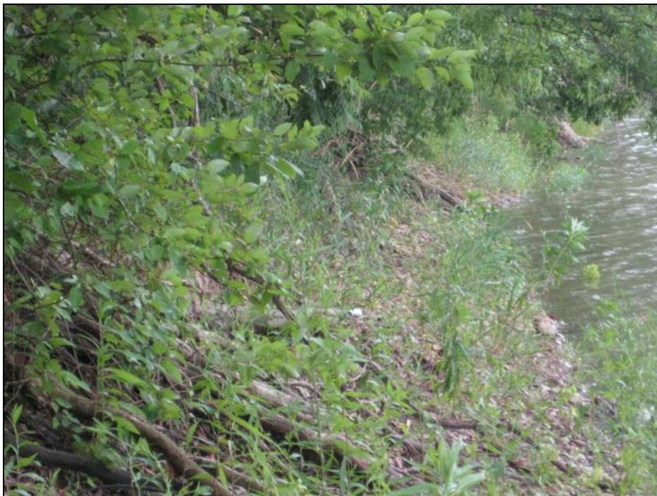
Photo 2. Toe of the Embankment, Showing Well Developed Root Mass and the Weathered Upper Surface of the Sevier Shale
